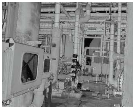
▲ Realistic looking, gray-scale scan images of plant interiors are characteristic results from phase-based scanners—Image courtesy: BE&K
